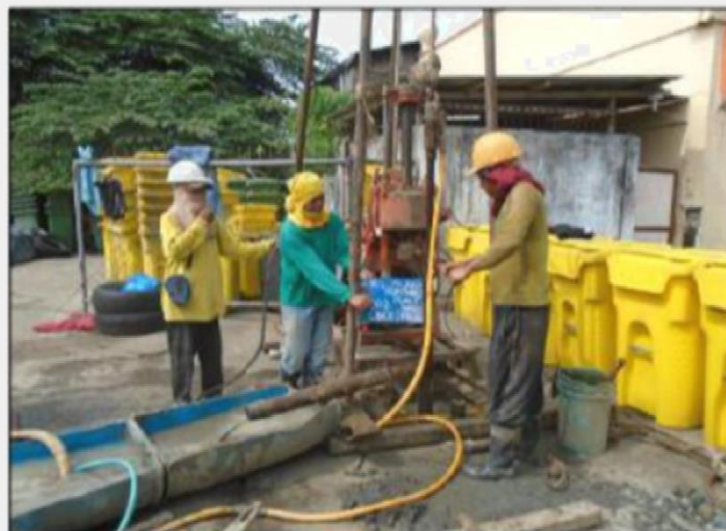
Figure 3-3. Actual Borehole Location & Drilling Activity
