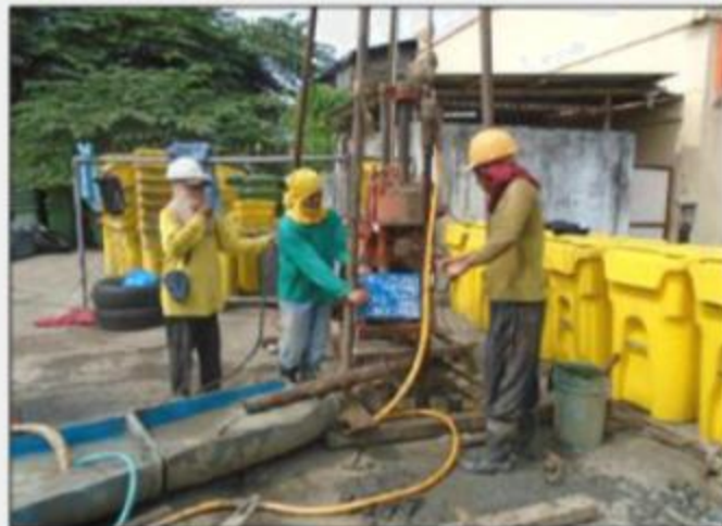
Figure 3-3. Actual Borehole Location & Drilling Activity
