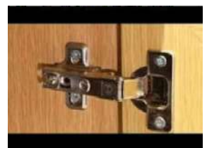
TYPICAL DETAIL OF CONCEALED HINGES
