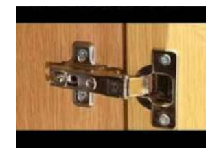
TYPICAL DETAIL OF CONCEALED HINGES
