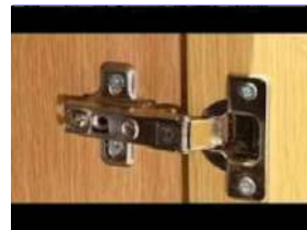
TYPICAL DETAIL OF CONCEALED HINGES
