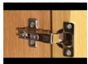
TYPICAL DETAIL OF CONCEALED HINGES
