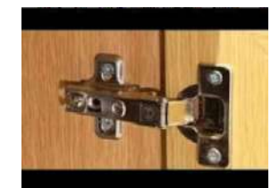
TYPICAL DETAIL OF CONCEALED HINGES
