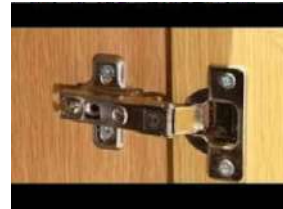
TYPICAL DETAIL OF CONCEALED HINGES
