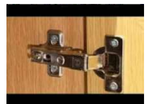
TYPICAL DETAIL OF CONCEALED HINGES
