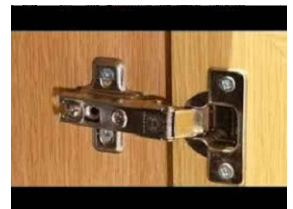
TYPICAL DETAIL OF CONCEALED HINGES
