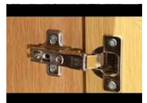
TYPICAL DETAIL OF CONCEALED HINGES
