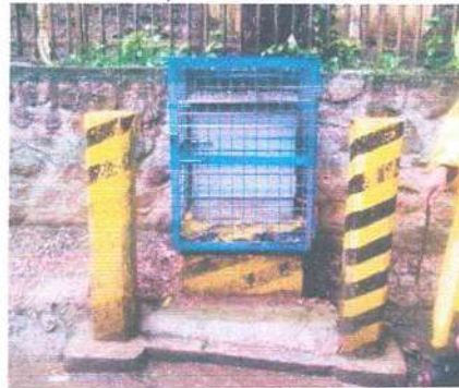
Picture-1. Sample enclosure with barricade
