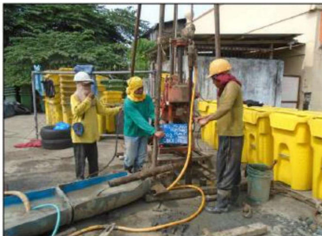
Figure 3-3. Actual Borehole Location & Drilling Activity
